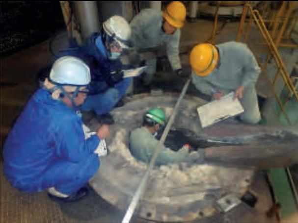
Technical training: break out lining material with the customer, identification of lining failure
