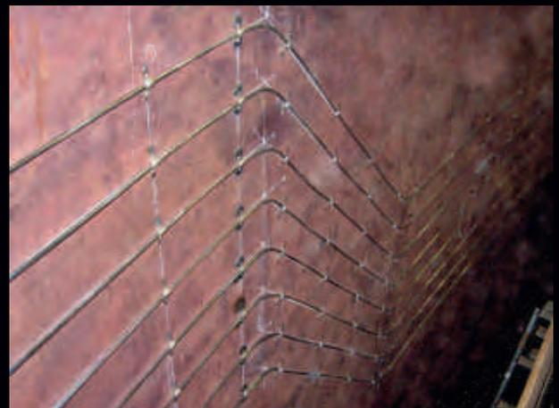
OPTISAVE installation on the inside of a water-cooled submerged arc furnace
