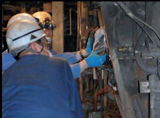
Tear out and confirmation of displayed wear on the channel furnace
